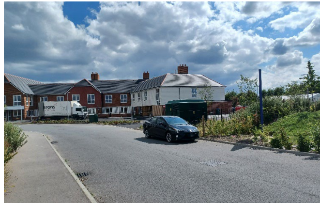
Care home to south
